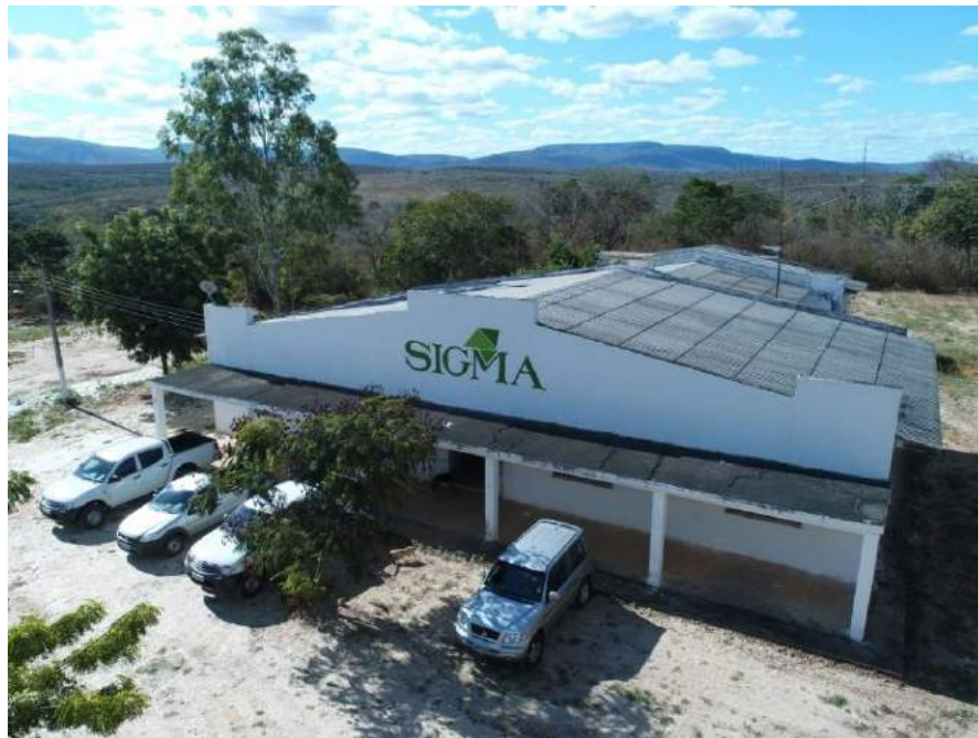
Figure 5-2: Field Office (location 6 in Figure 5-2)
